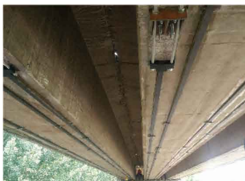
土木工程加固 Civil engineering reinforcement
