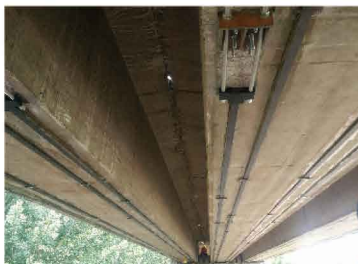
土木工程加固 Civil engineering reinforcement
